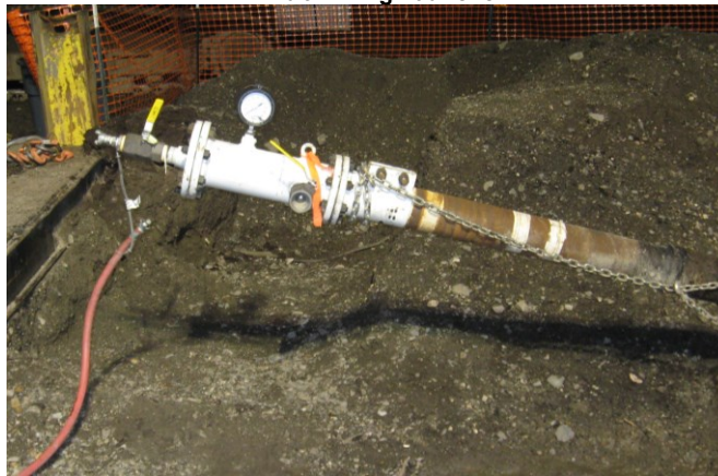
Exhibit 12- Pig Launcher
