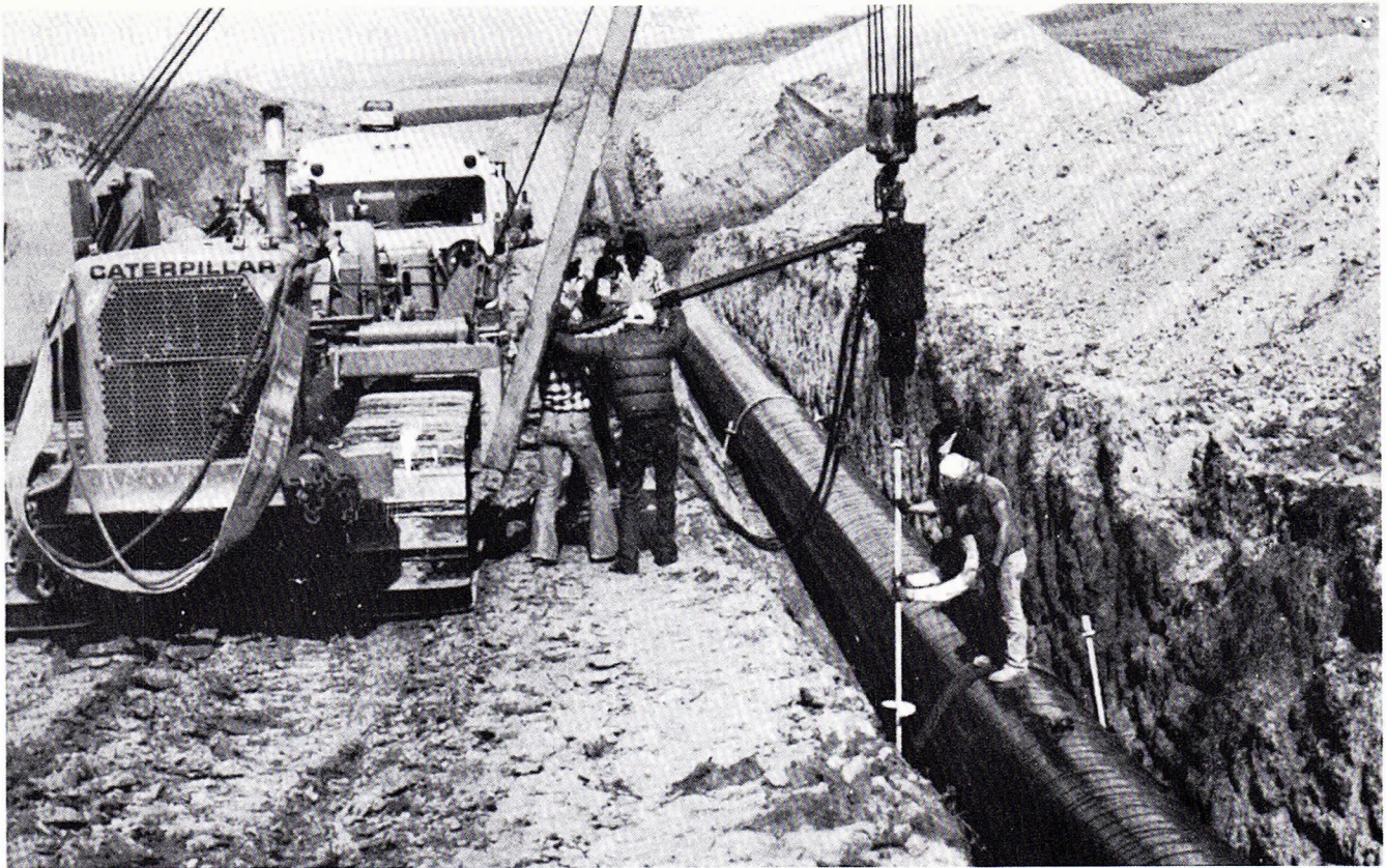
Technique of setting anchors using a sideboom tractor (Fig. 1).
