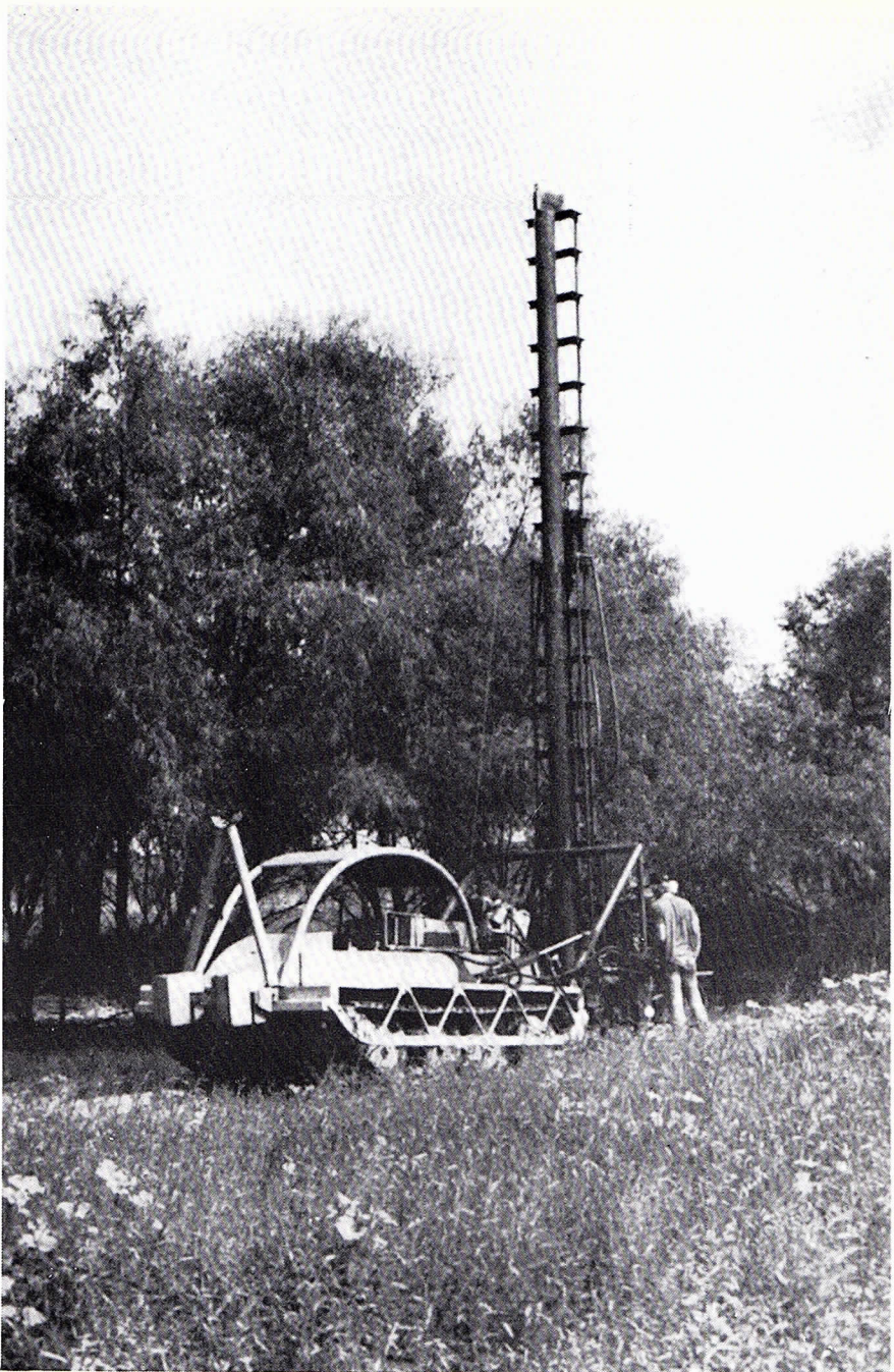
Bombardier vehicle equipped with a boom being used for installing and testing full-size auger anchors (Fig. 2).
