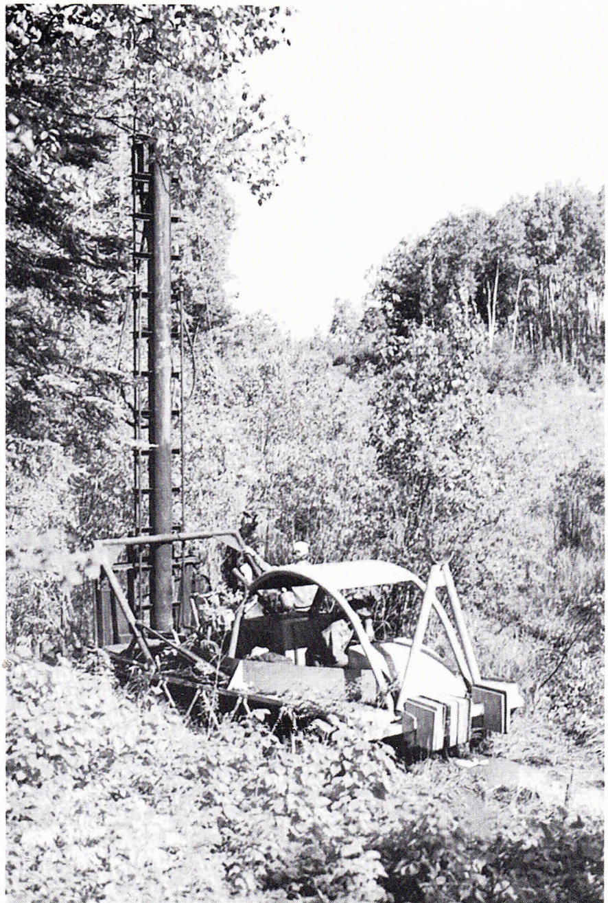
Wet footing. Bombardier muskeg tractor crosses wet areas in making soil survey in Minnesota swamps. Vertical boom carries hydraulic powered drill.
